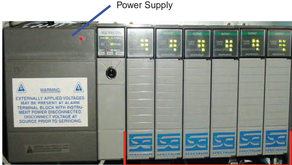
4-20mA Output Modules (6X)
